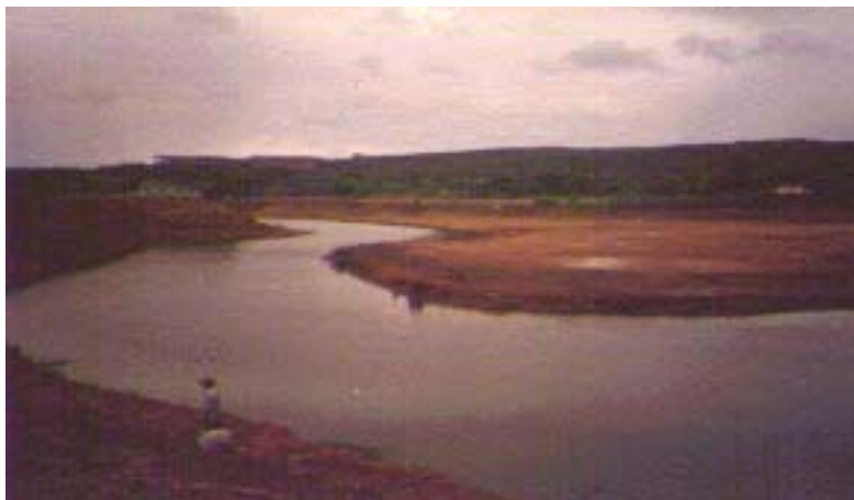
Plate. 5.1 Deepening and widening of spill channel r.
