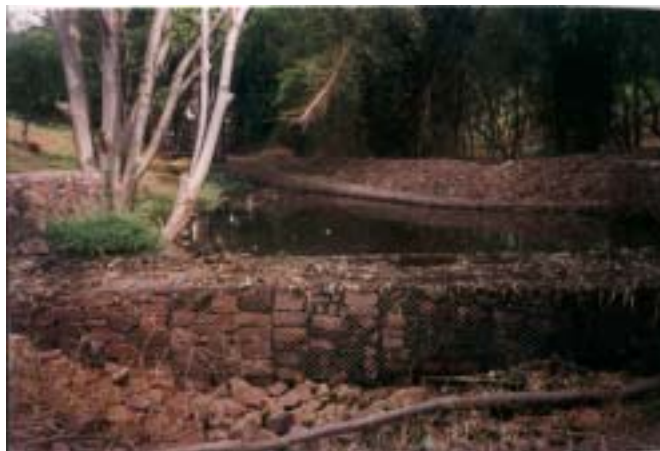
Plate 5.3. Gabien structure near Lower Lake
